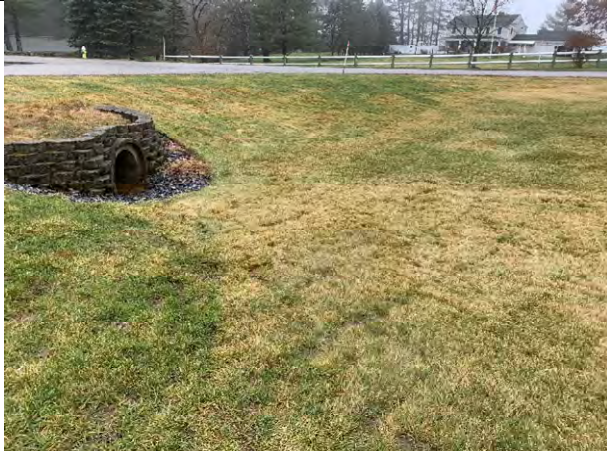
29 Gundalow - 1 (Drainage Area)
