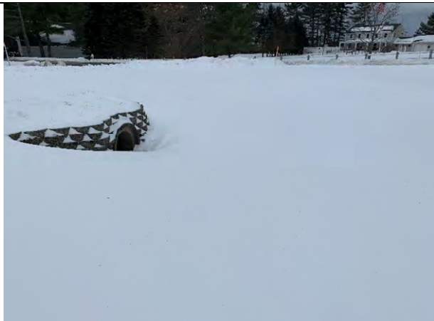
29 Gundalow - 1 (Drainage Area)
