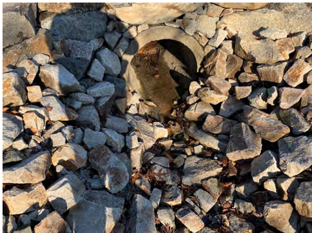
64 Gundalow - 1 (Drainage Course)
