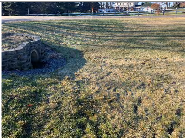
29 Gundalow - 1 (Drainage Area)
